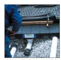
All Center and Side Track Pans are molded with pipe fitting locators at their lowest point. Below-grade piping can be installed to channel large spills to oil/water separators, holding ponds, etc.
